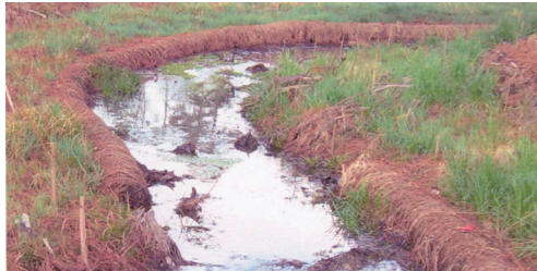
Figure 6.72b Coir log installation, NC Ecosystem Enhancement Program
