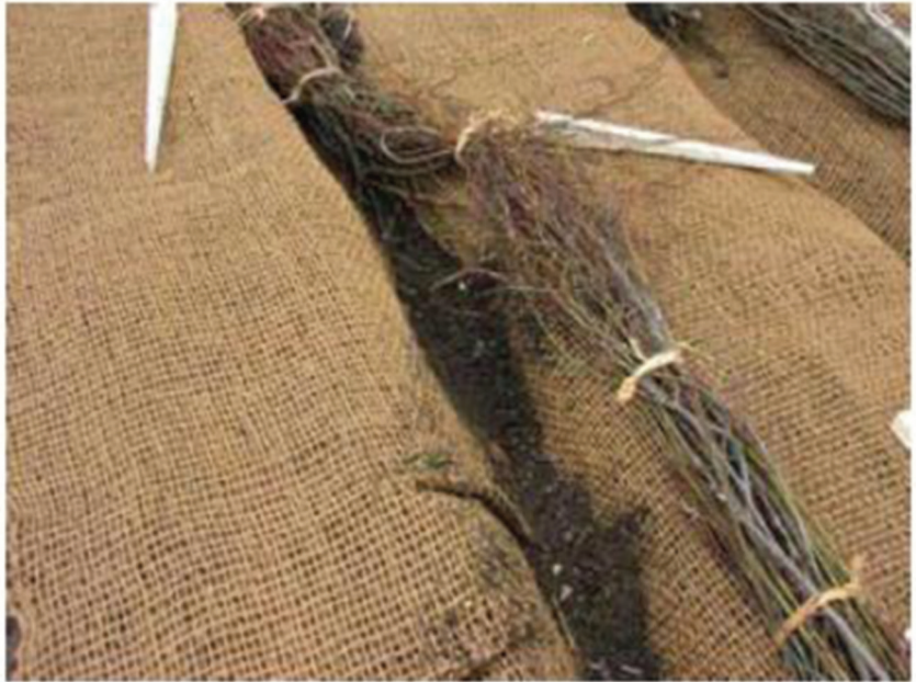
Figure 6.72c Combining fascines and fabric
