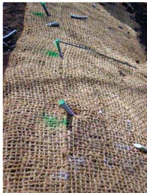
Figure 6.72d Live cuttings installed in fabric
