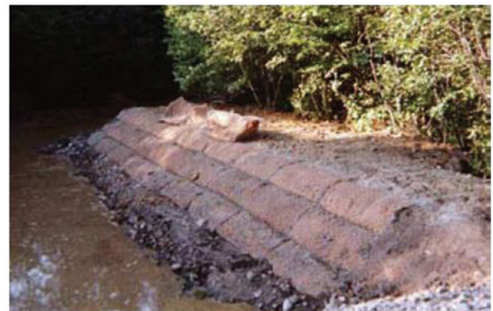
Figure 6.73e Vegetated gabions under construction
