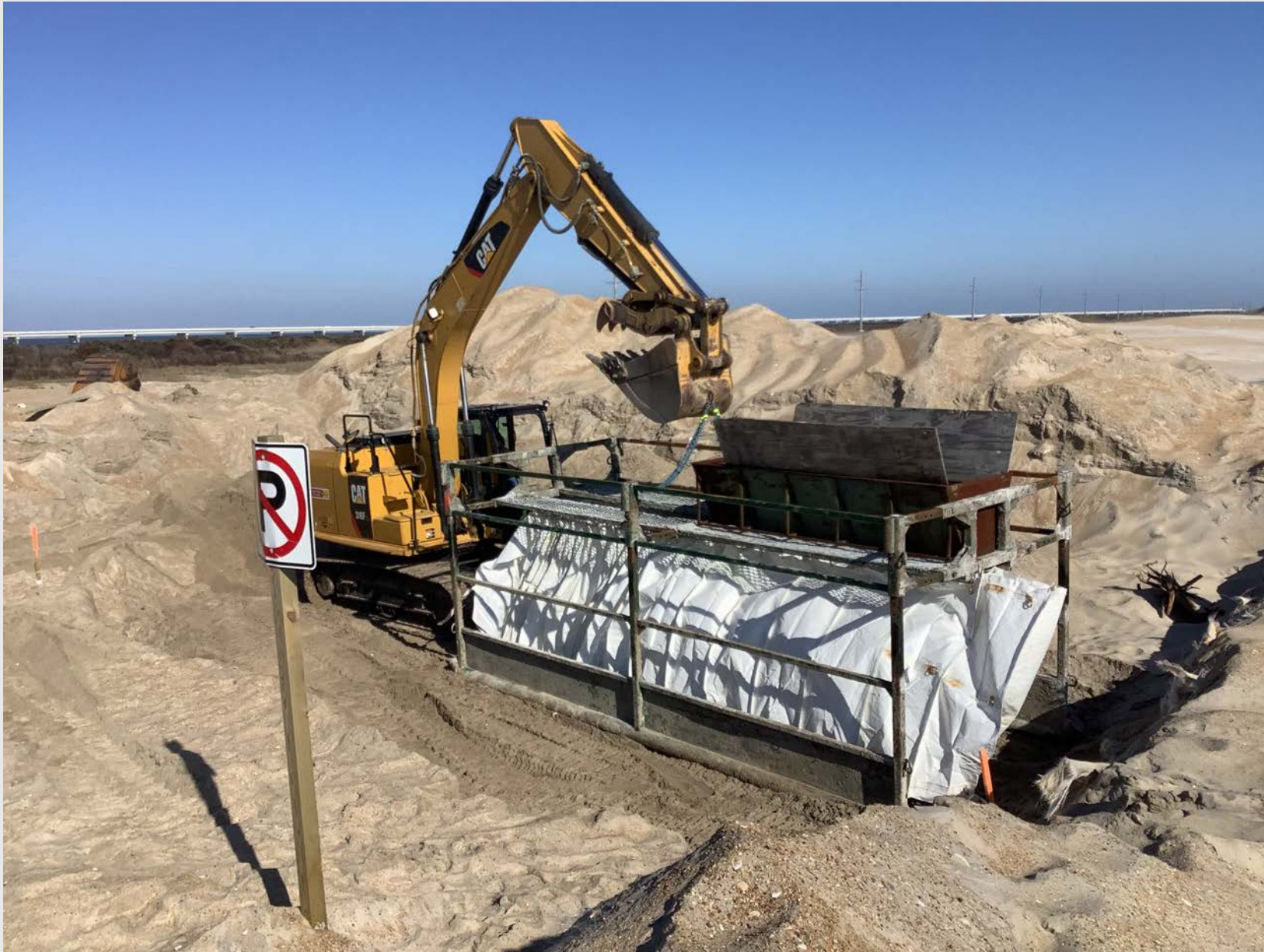
Installation of PermaShield sandbags at Mirlo Beach.
