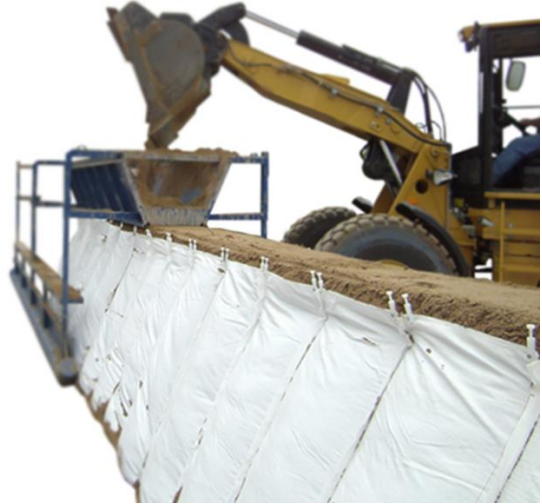
Illustration I: Installation Platform for concrete for quick and efficient fill.
