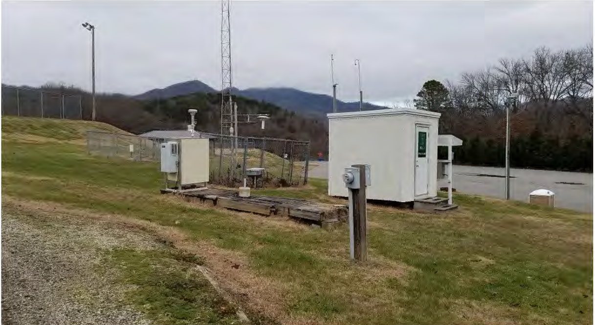
Figure 10. The Bryson City ozone and particle monitoring site
