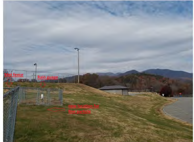
Figure 100. Looking northwest at the new location
