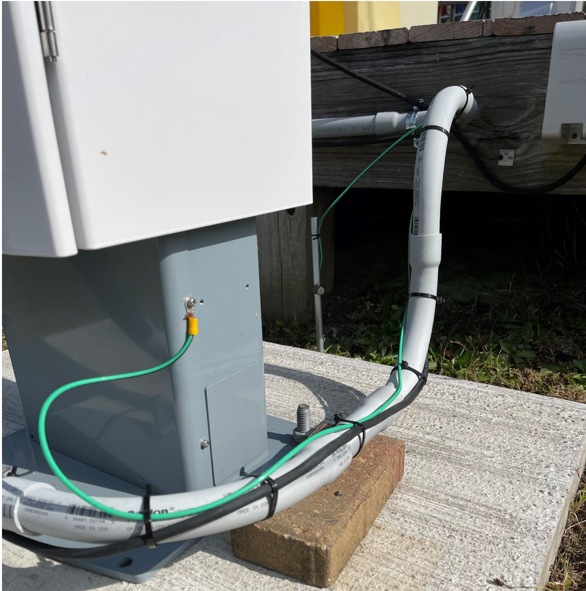
Figure 18: Vaisala CL-51 External Ground Depiction
