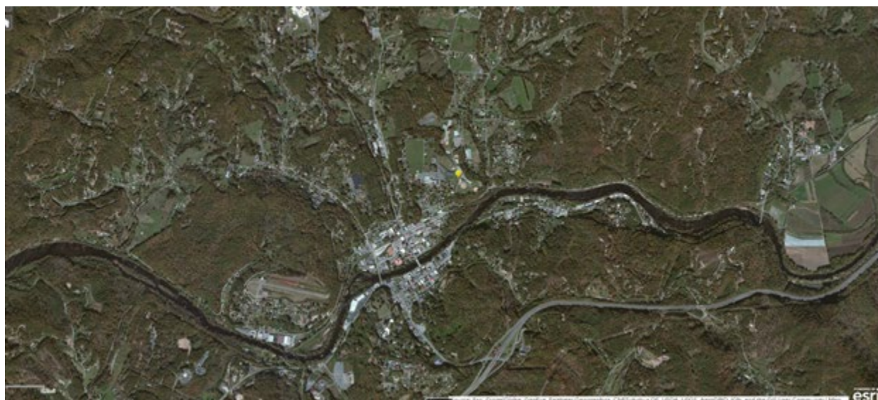
Figure 20. Aerial View of Bryson City Site
