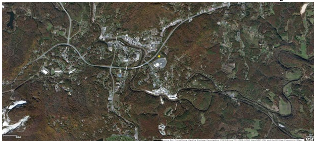
Figure 15. Aerial View of Spruce Pine Site
