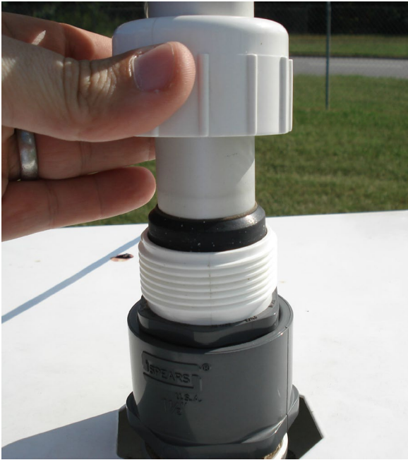
Figure 59. Inlet Tube Flange.
