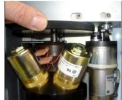
**Figure 43. Use the Wheel to Raise and Lower Solenoid Manifold**
