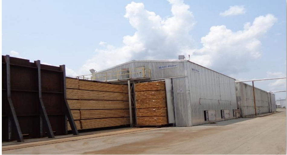
Figure 5-2: Continuous Lumber Drying Kiln (Double Track Arrangement - Cross-sectional View)
