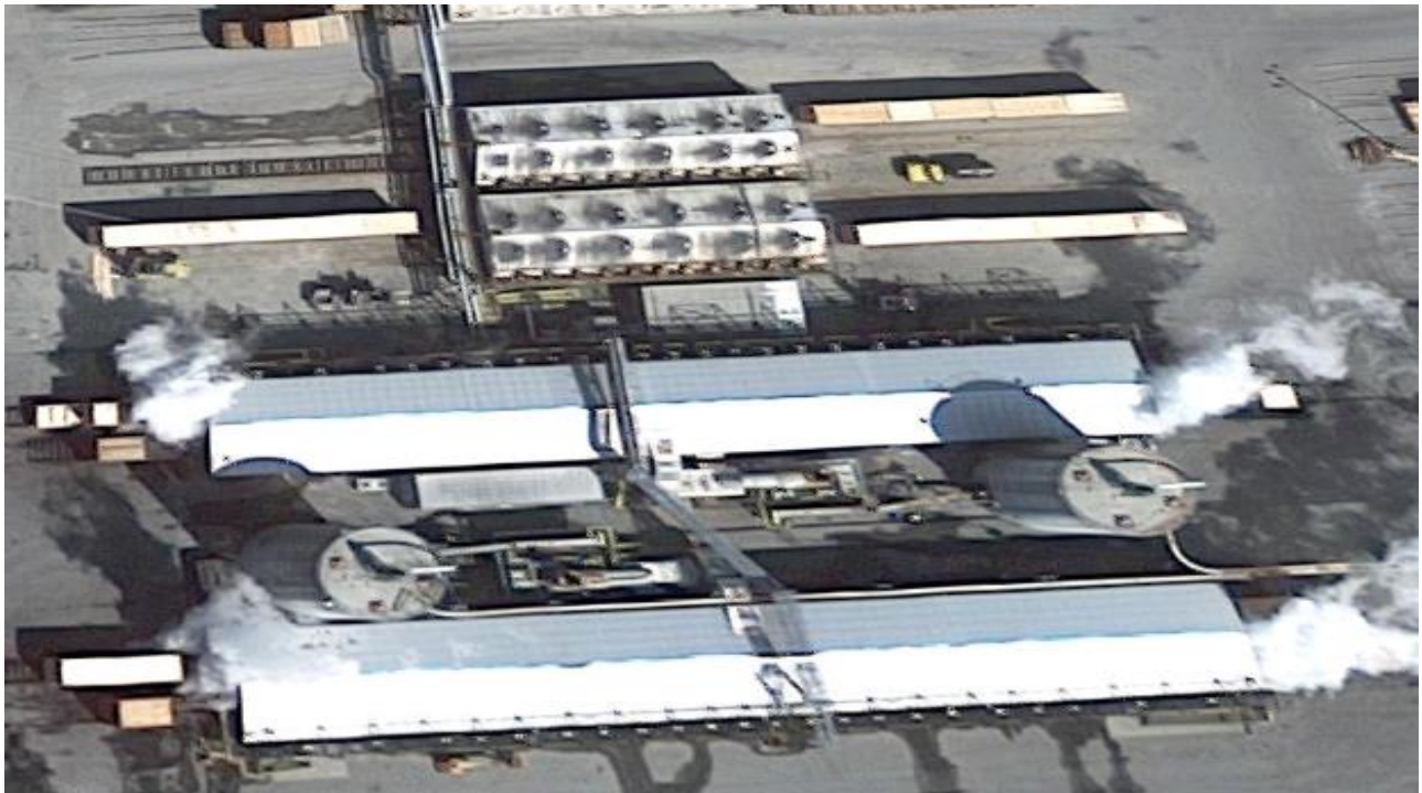
Google Satellite 3D image of the two steam-heated batch kilns (top middle), two continuous direct-fired kilns, and two fuel silos.
