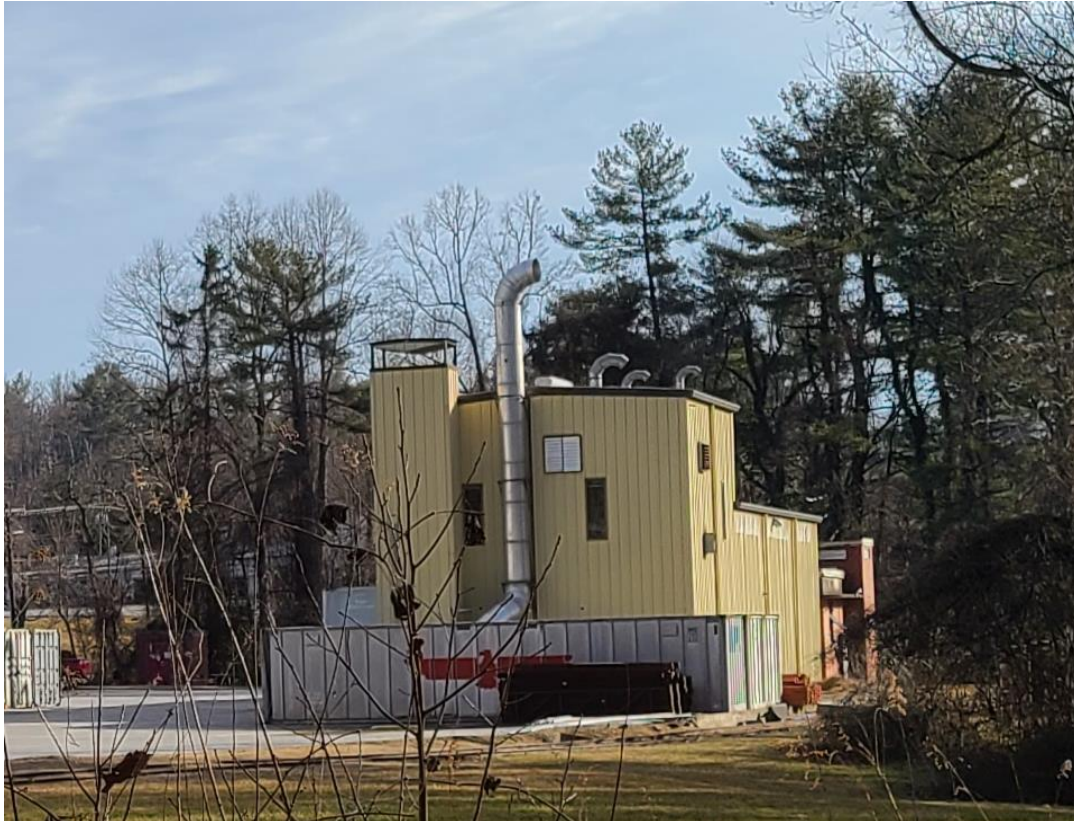
Figure 2: BCI process building (from most recent inspection report)
