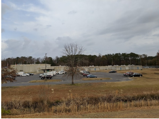
Figure F5. Pitt Co Ag Center site looking north
