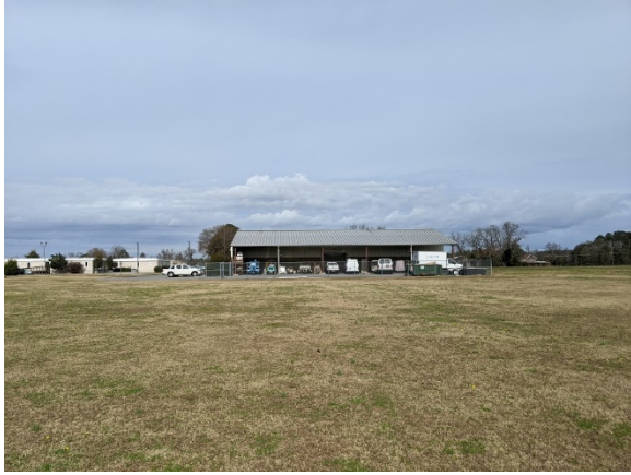
Figure F30. Looking north from the LCC site
