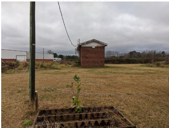
Figure F16. Looking west from the Jamesville site
