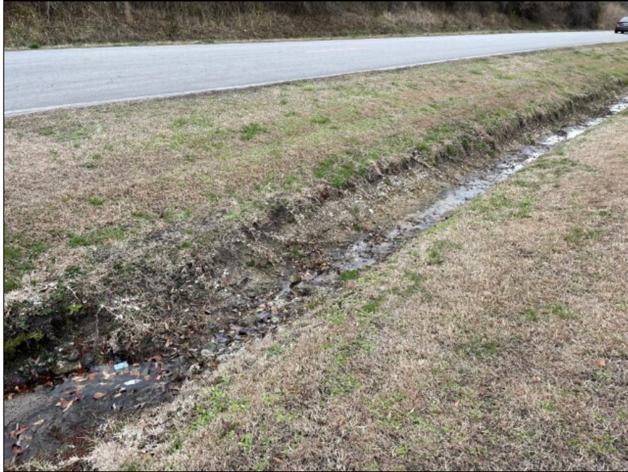
3 - View of drainage ditch along Neals Creek Road
