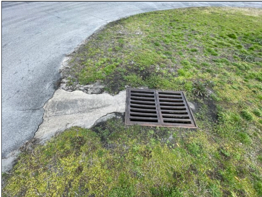
2 - View of storm drain on the eastern portion
