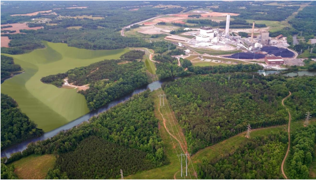
Active Ash Basin Post Closure View
