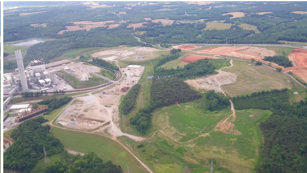
Current View of Unit 5 Ash Basin
