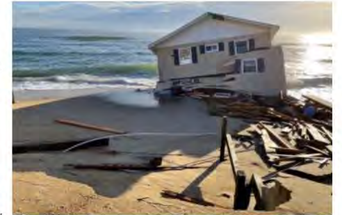
Collapsed home in Rodanthe. (File photo: National Park Service)
