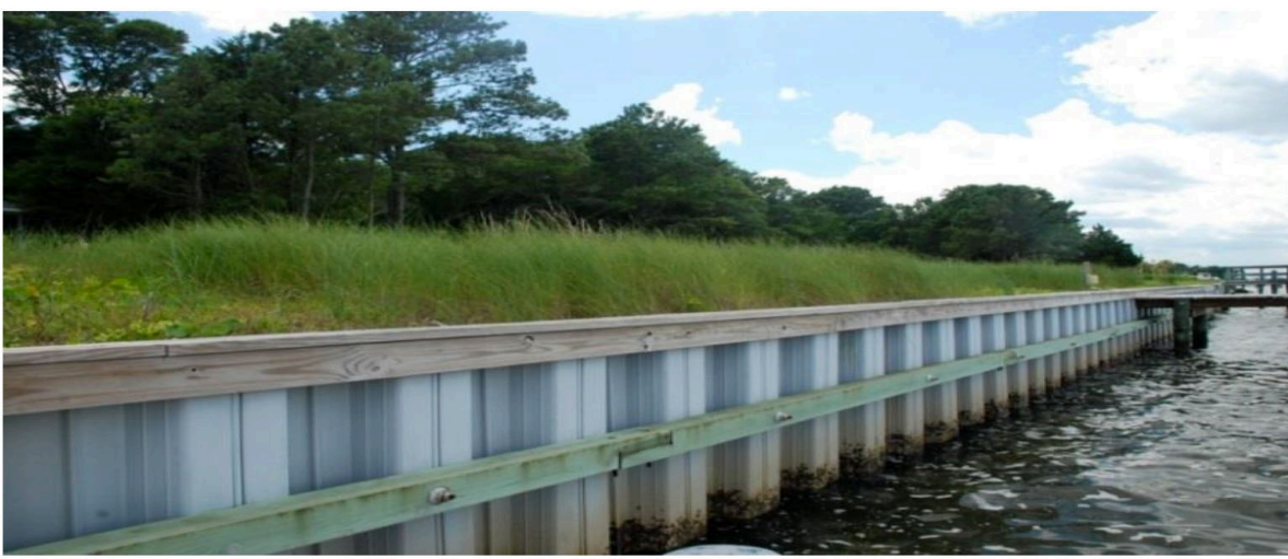
Bulkhead constructed using vinyl, Pivers Island, N.C.
