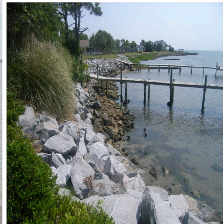
Riprap revetment with grasses and lawn, N.C.
