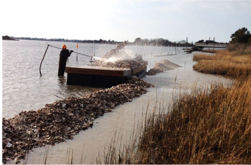
Loose oyster shell sills during construction
