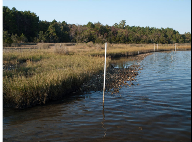
Loose oyster shell sill after Hurricane Matthew
