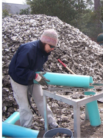
Step 2: Pull bags over PVC tubes
