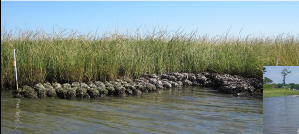
Marsh toe revetment
