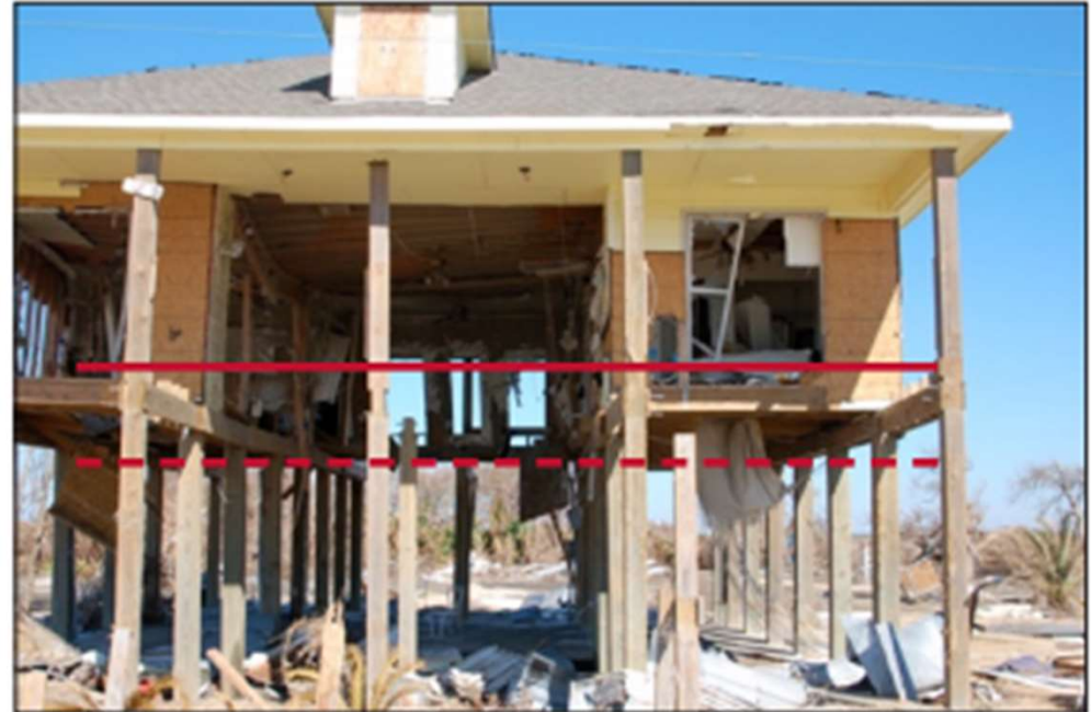
Figure 2. Bolivar Peninsula, TX, V-zone house constructed with the lowest floor (bottom of floor beam) at the BFE (dashed line). The estimated wave crest level during Ike (solid line) was 3 to 4' above the BFE at this location.
