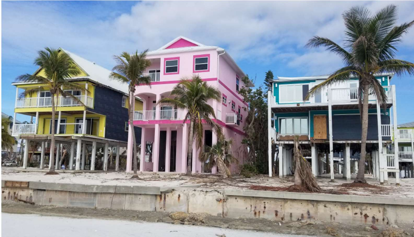
Figure 1: Three neighboring buildings with varying degrees of elevation and damage on Fort Myers Beach, Florida, after Hurricane Ian. The right-most building has the lowest elevation of the three and the most damage to the lower levels, whereas the middle building has the highest elevation and minimal damage to the lower levels.
