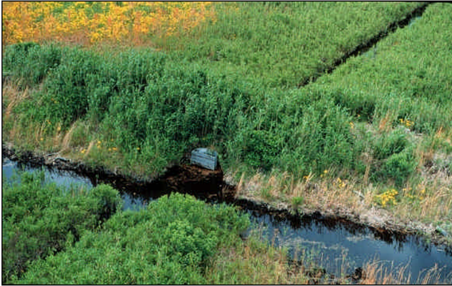
Figure 25. Example of a water control structure along a drainage ditch.
