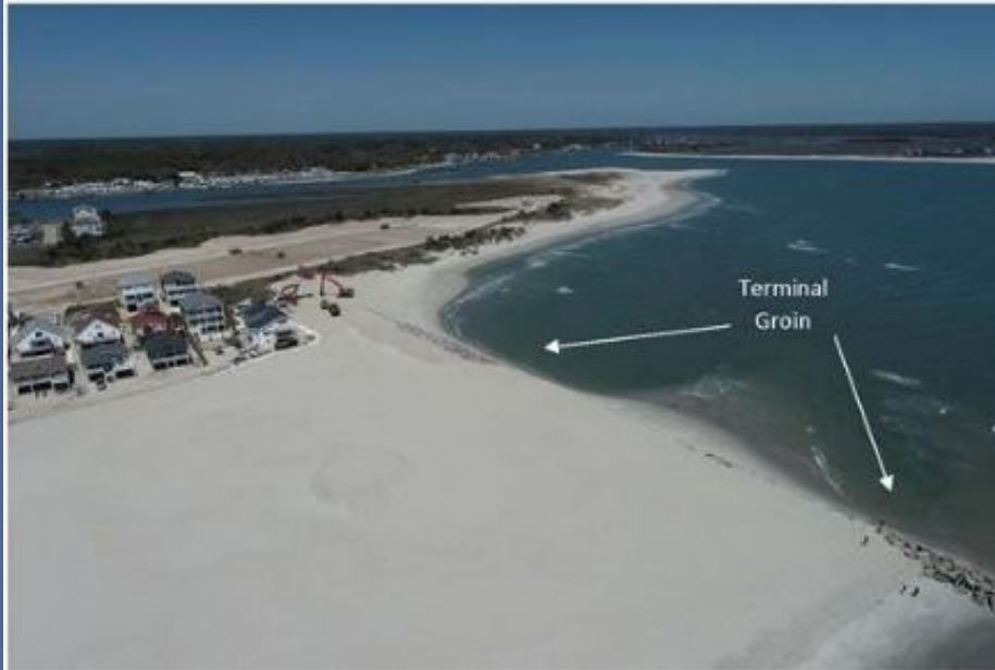
After Construction: Facing northeast on 4/11/22
