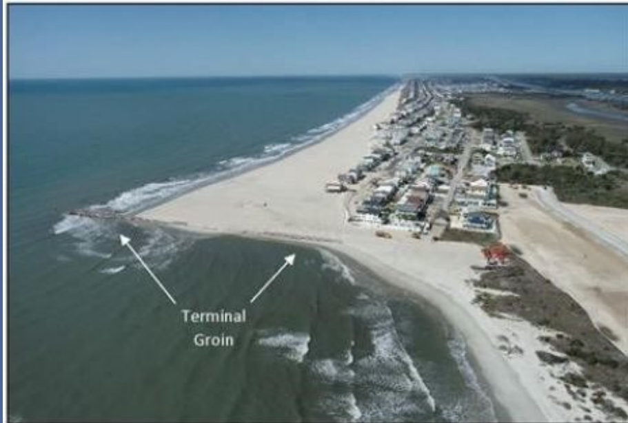
After Construction: Facing west along Ocean Isle Beach's east end on 4/8/22
