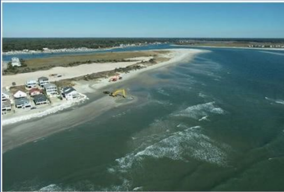
Before Construction: Facing northeast on 11/16/21
