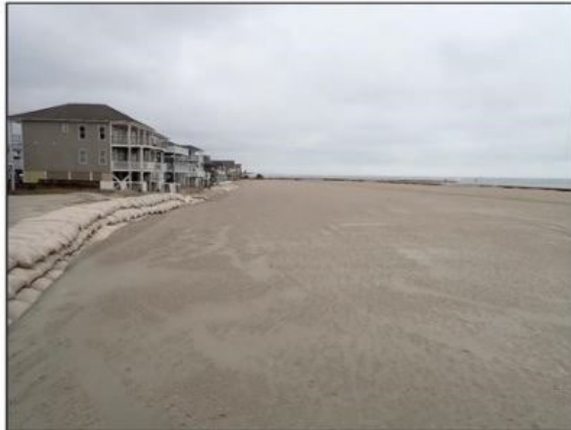
After Construction: Facing east at Shallotte Blvd. on 4/8/22
