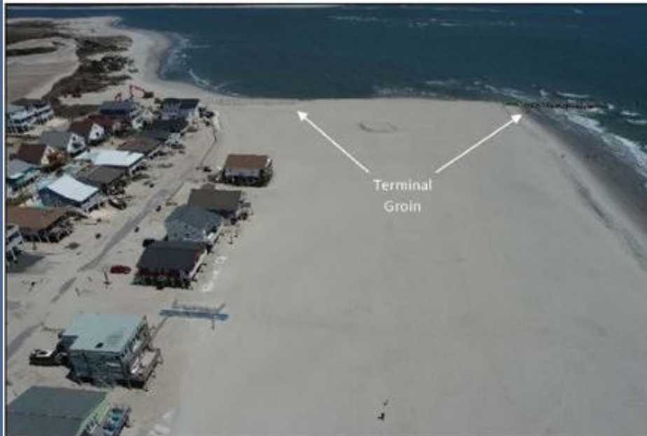
After Construction: Facing east from above Columbia St. on 4/11/22
