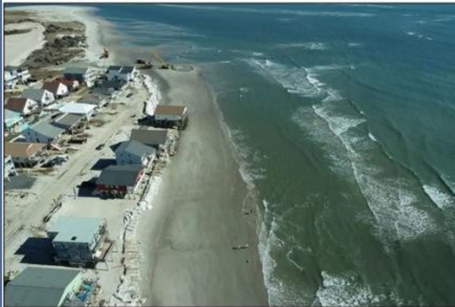
Before Construction: Facing east from above Columbia St. on 11/16/21
