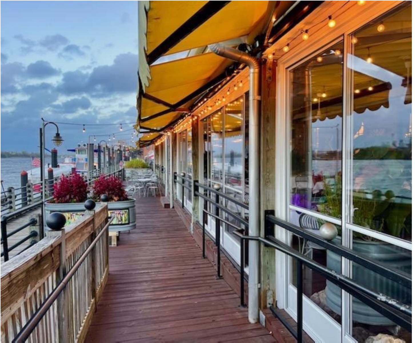
West Wall Enclosure
