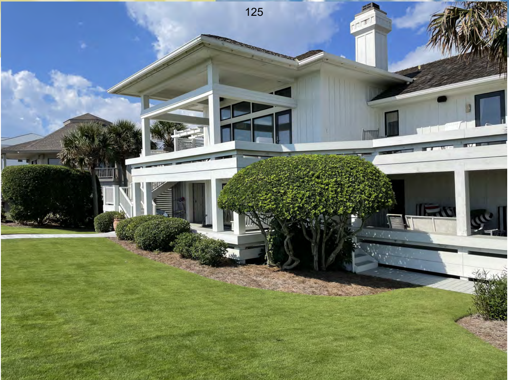
View of existing residence from ocean side facing west
