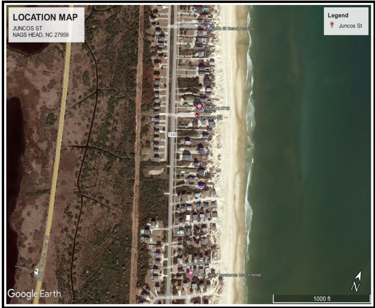
Figure 2. Location map displaying the proposed site location for the Juncos Street Dune Infiltration System
