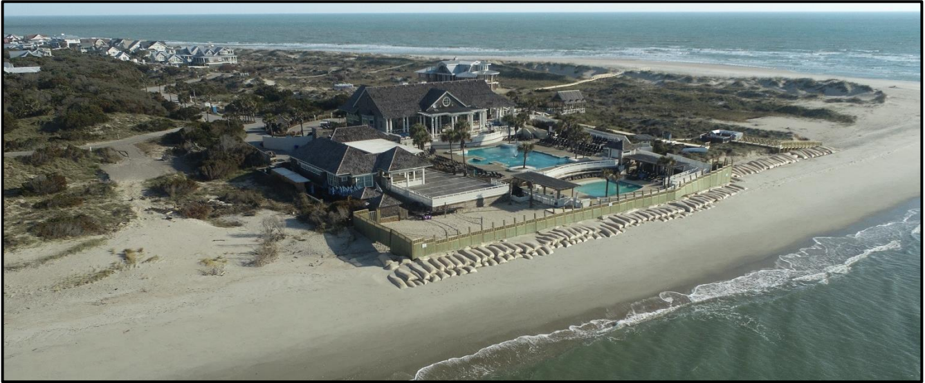
Figure 6: Drone imagery from November 1, 2022, 6-months post-installation of the sandbags. Note the height of the bags relative to the top of the wooden fence. Image courtesy of Olsen Associates, Inc.
