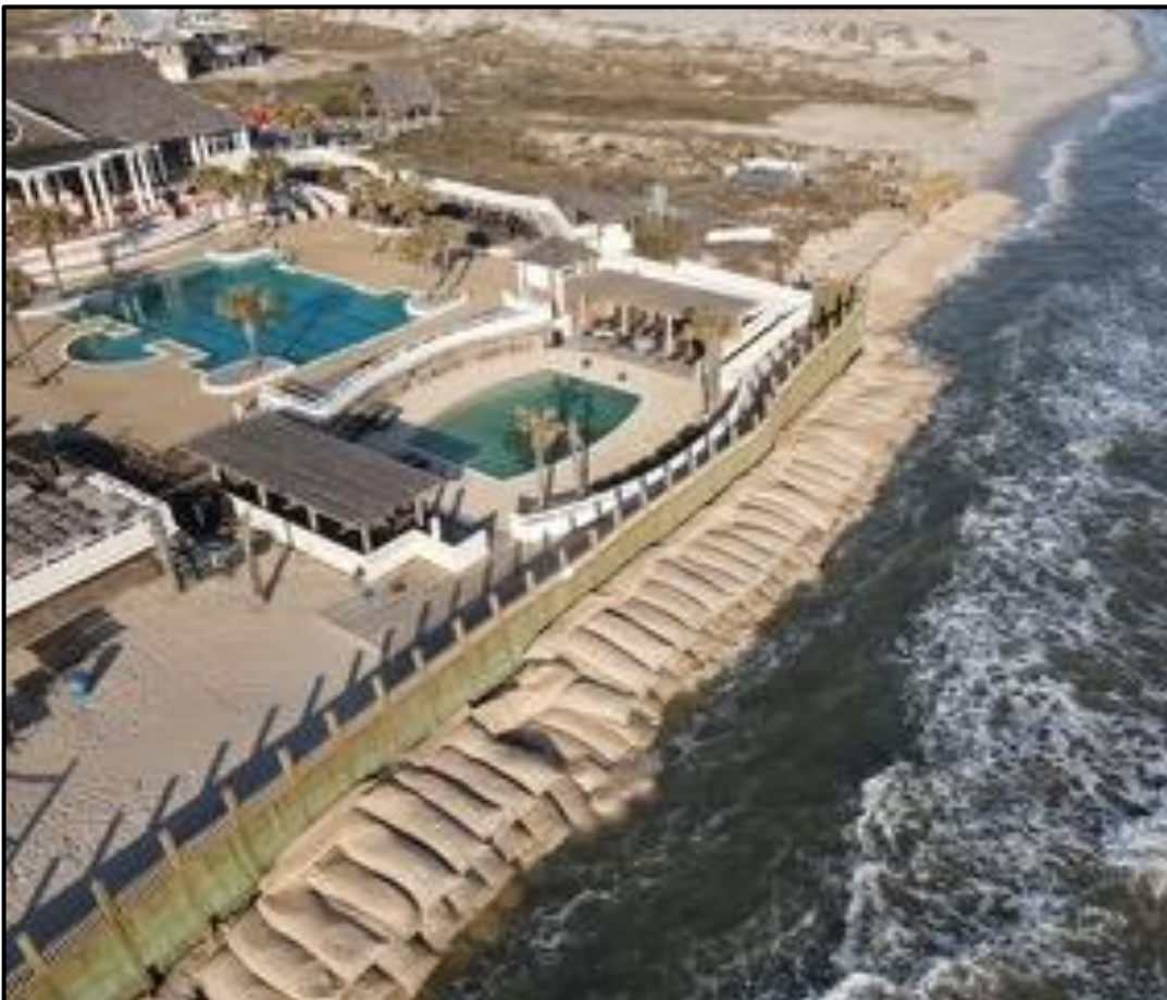
Figure 7: March 2023 drone imagery of a high-water event impacting the sandbags approximately 10-months post-installation. Image courtesy of the Shoals Club.
