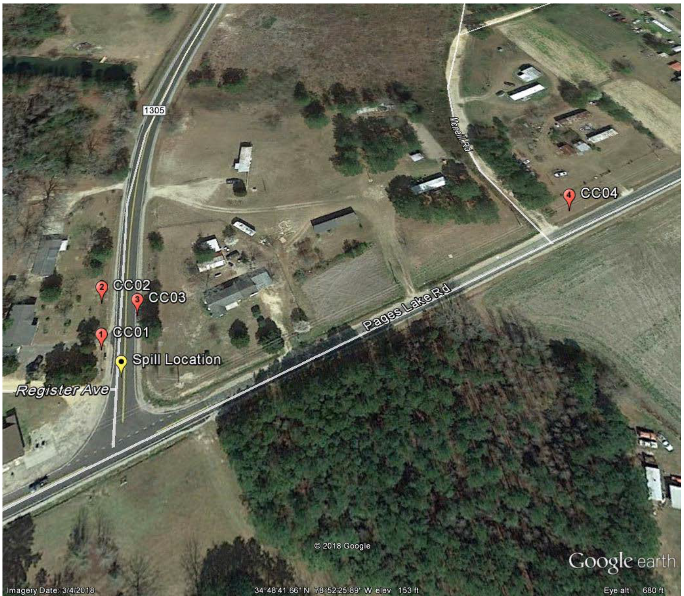
Investigation of liquid spilled from a truck transporting material for Chemours on 9/18/18. Figure 1.
