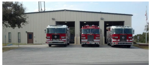
NTB Fire Department – Station 1 Image Source: Town of North Topsail Beach.
