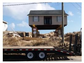
Retrofitting of an existing oceanfront home through elevation. *Image Source: HCP*.
