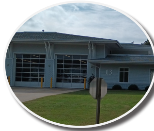
Public Infrastructure and Services
