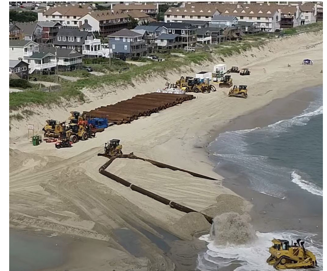
Beach renourishment was conducted for approximately 3.97 miles of shoreline from Southern Shores / Kitty Hawk town line to Kitty Hawk / Kill Devil Hills limits from August to October of 2022 at a cost of $9,600,000.
