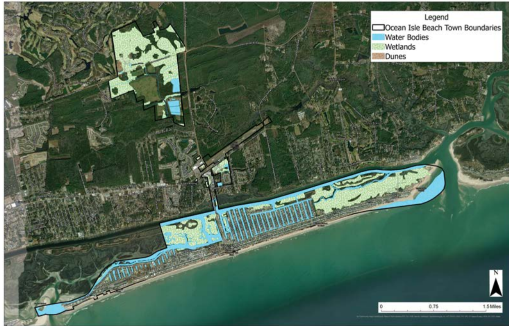
Figure 3. Natural infrastructure within the Town of Ocean Isle Beach.
