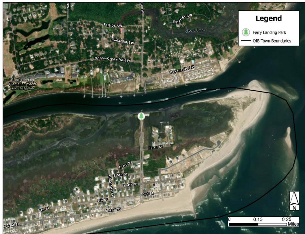
Figure 4. Ferry Landing Park, potential site for a living shoreline demonstration project.
