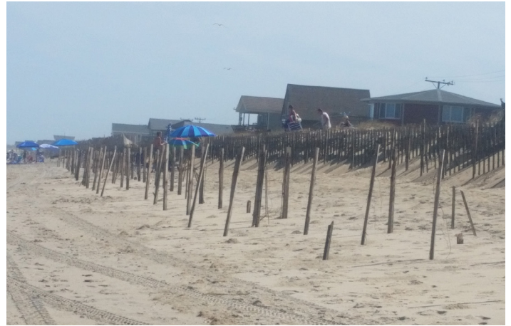
Dune erosion from Hurricane Dorian in 2019
