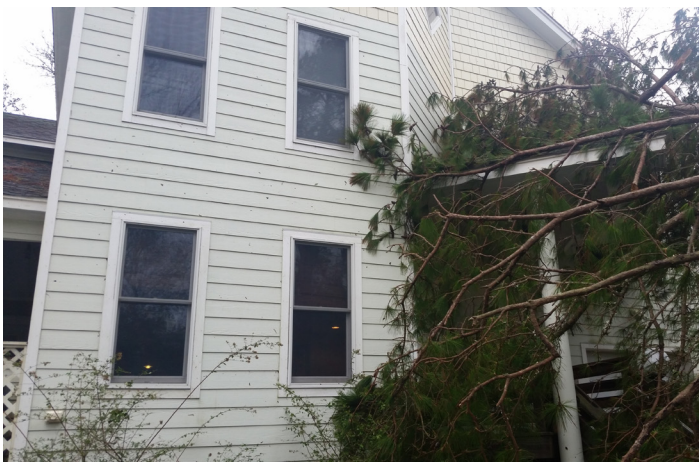
Fallen tree from Hurricane Matthew in October 2016
