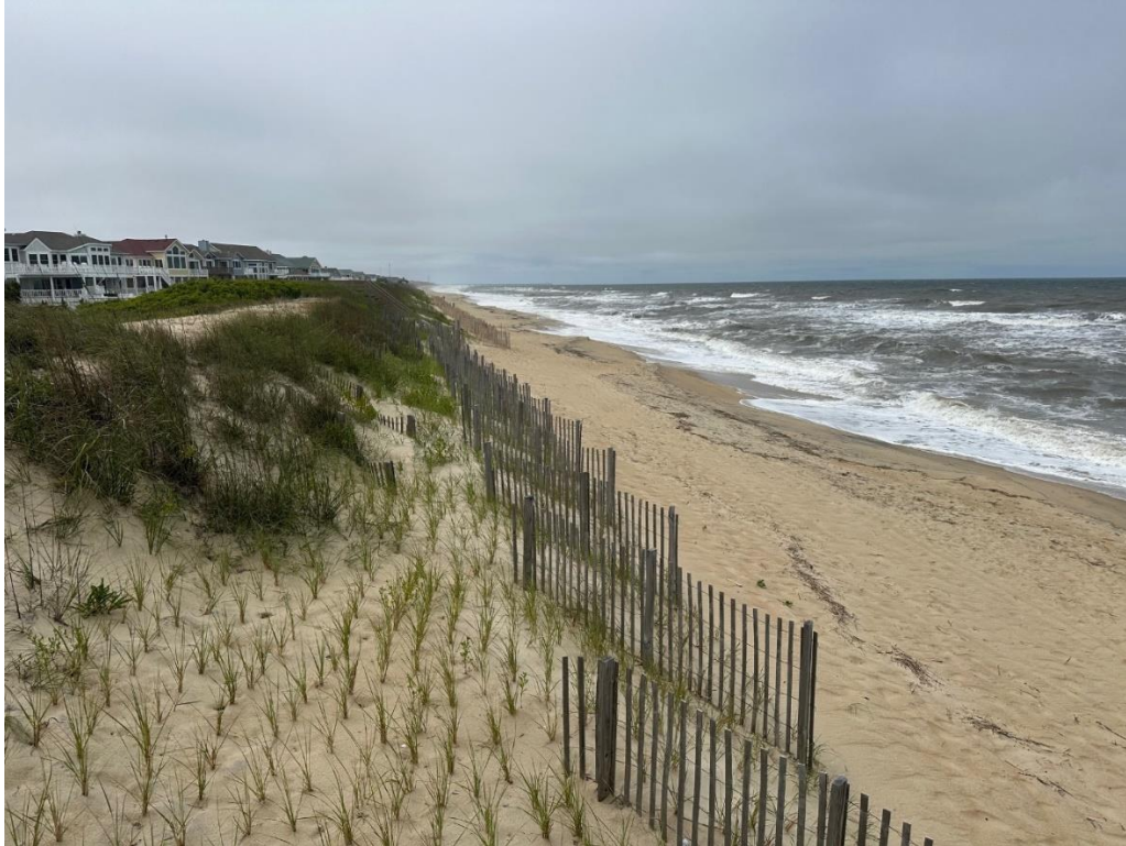
Figure 1. A typical wooden sand fencing installation.
