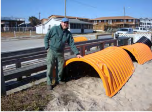
Figure 5. An example of the type of chamber that can be used for the DIS.
