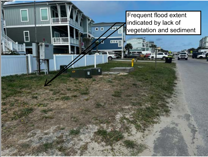
Photo 14: Frequent flooding extends to sanitary sewer pump station at intersection of Ocean Dr and Sherrill St. Note change in development from 2020.
