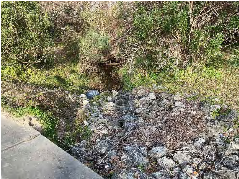
Photo 10: Ex. Outlet @ Womble St. and Elizabeth Dr. View looking North-East.
