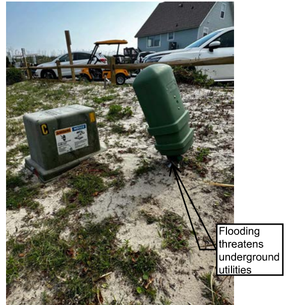
Photo 17: Sand deposition indicates flooding extends to utility boxes. Some appear to be in substandard condition.
