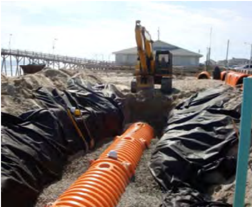
Figure 7. Installation of a DIS at Kure Beach, NC.
