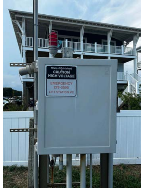
Photo 17: Sand deposition indicates flooding extends to utility boxes. Some appear to be in substandard condition.
