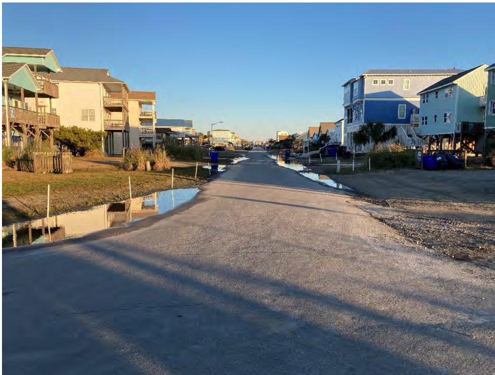
Photo 16: Site 3 area @ 79 th St. and Ocean Drive. View of ponding looking South-East.
