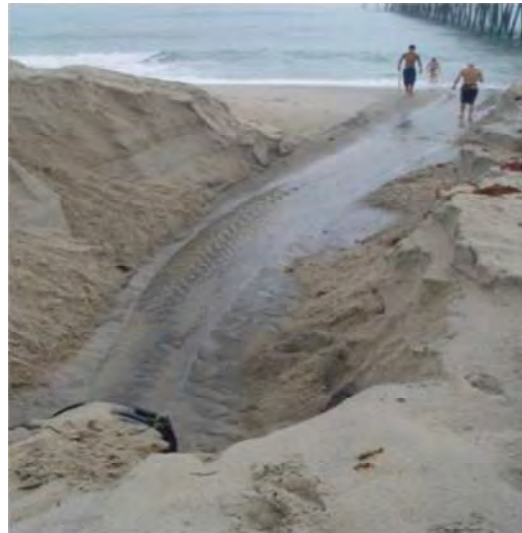
Figure 4. Despite warnings, contact with discharging stormwater often still occurs.
