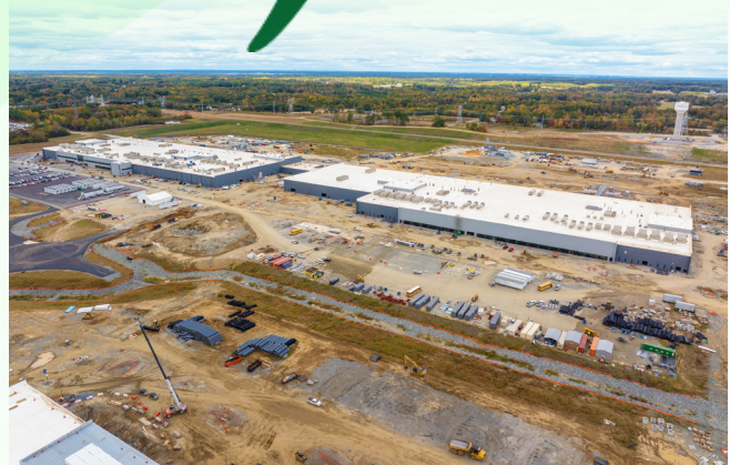
Construction at the North Carolina Battery plant in Liberty.
