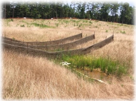
Figure 12 - Good Vegetative Stabilization
