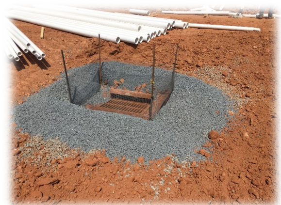
Figure 13 - Good Inlet Protection
