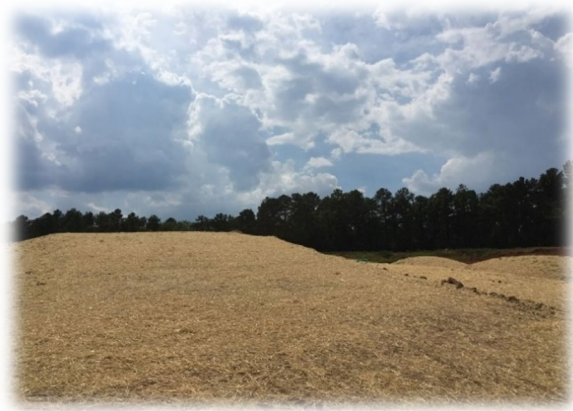
Figure 9 - Good Application of Ground Cover
