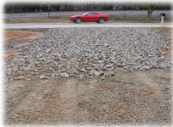
Figure 7 - Good Construction Entrance
