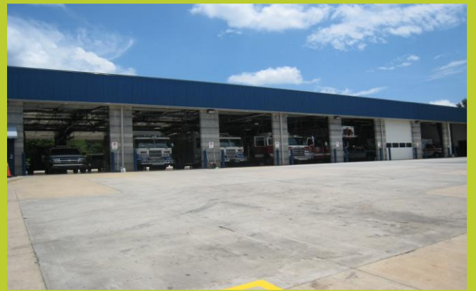
The size of Skyland Fire Department's facility allows it to inspect, service, and house fire engines from other regional departments.
