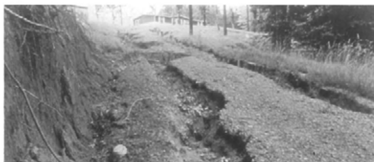
Bank erosion resulting from improperly protected land left void of vegetation.
