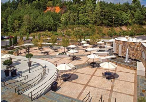
FIGURE 19: GREEN INFRASTRUCTURE AT A LOWE'S STORE IN WILKESBORO; HTTP://WWW.LANDSCAPEONLINE.COM/RESEARCH/LASN/2014/02/IMG/25194/25194-1.JPG
