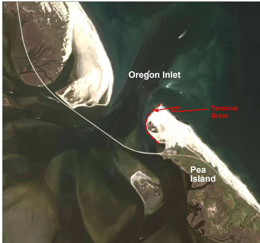
Figure II-23. Terminal Groin at North End of Pea Island
