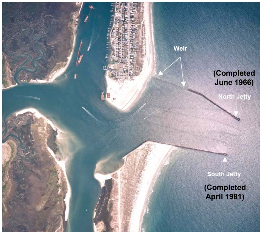
Figure II-19. Masonboro Inlet Jetties (May 2002 – USACE)
