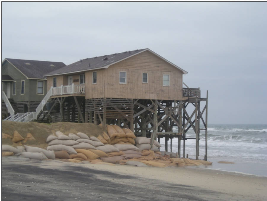
Figure II-21. Example of Sandbags Used as Temporary Erosion Control Structures at South Nags Head
