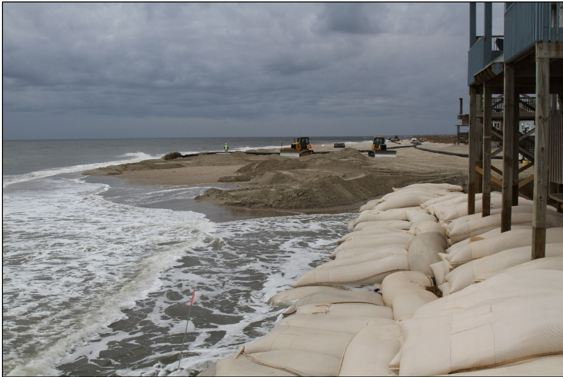
Figure III-62. Cutter Suction Dredge Operation (Oak Island)
