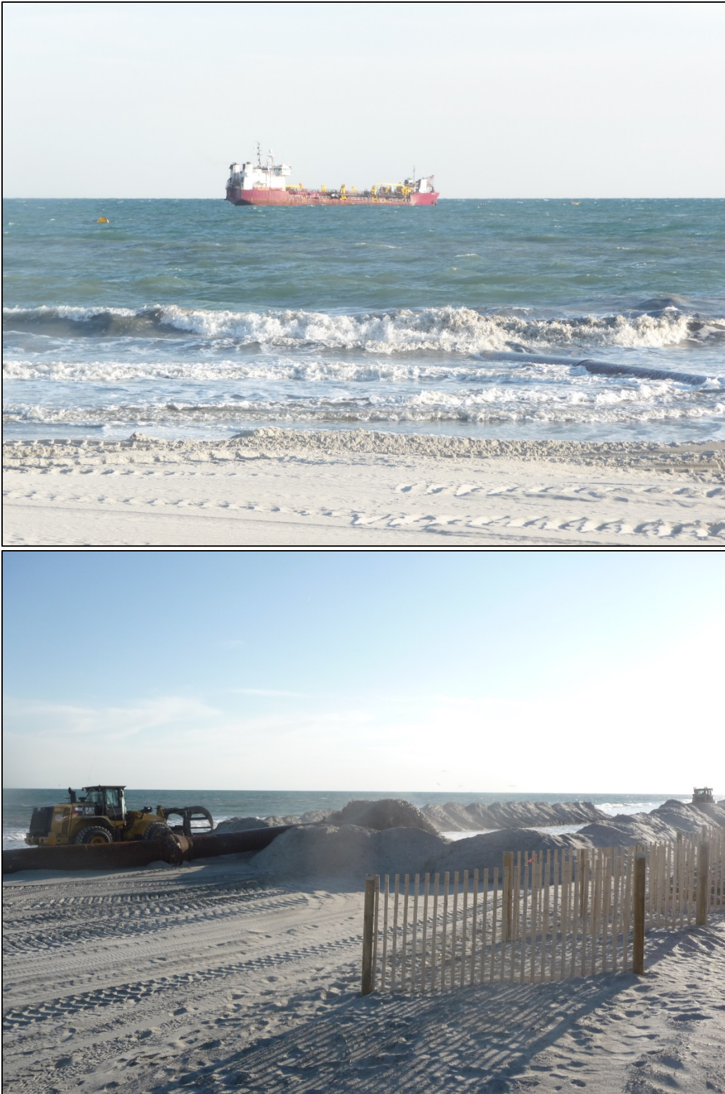
Figure III-63. Hopper Dredge Operation (Bogue Banks)
