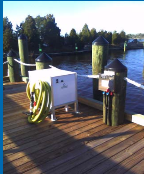
On Fixed Pier
