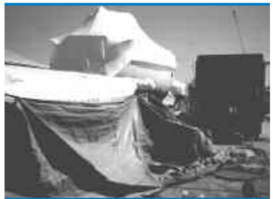
Boat enclosed for plastic media hull blasting.
