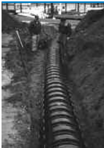
Infiltration chambers being installed.
