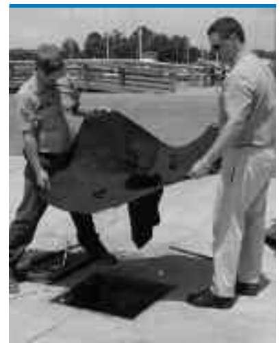
Inlet filter sock being installed.
