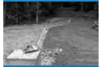
Level spreader constructed of concrete.
