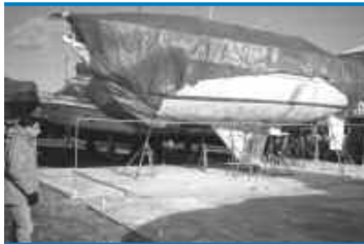
Concrete work pads are raised and surrounded by permeable gravel to control runoff.
