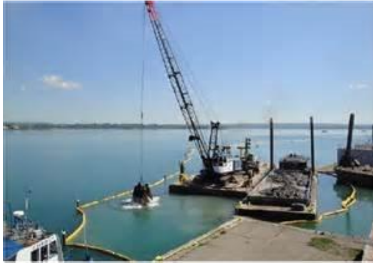
Figure 4. Photograph of Mechanical Dredging
