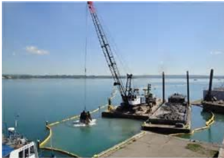
Figure 4. Photograph of Mechanical Dredging
