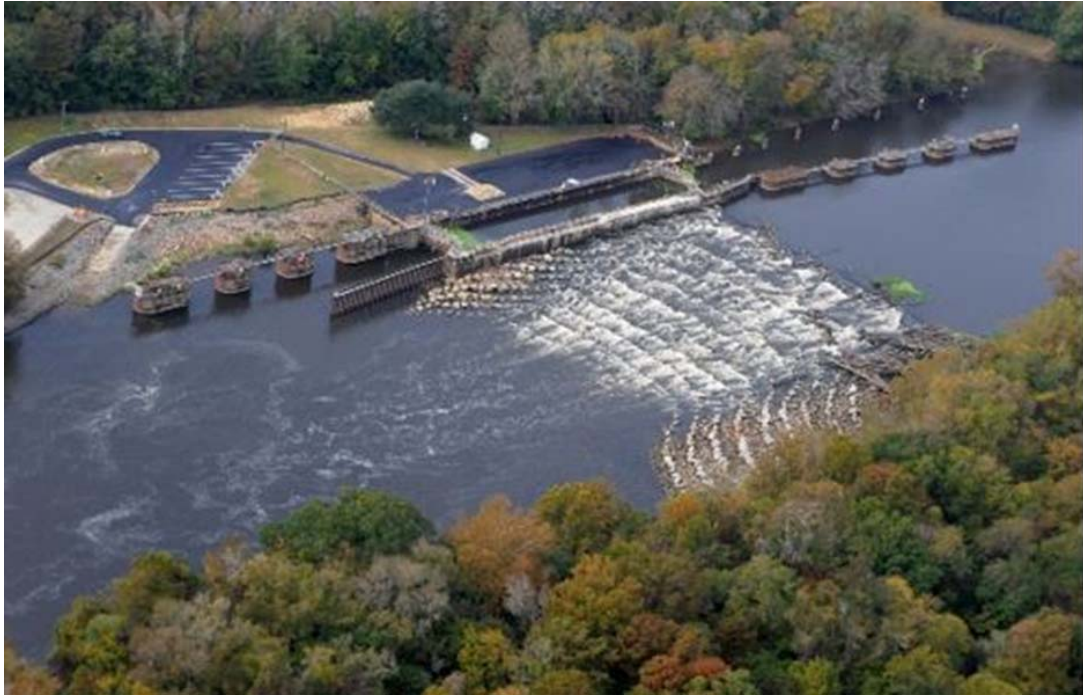
Figure 13. Photo of Existing Rock Arch Rapids Fish Ramp at Lock and Dam
