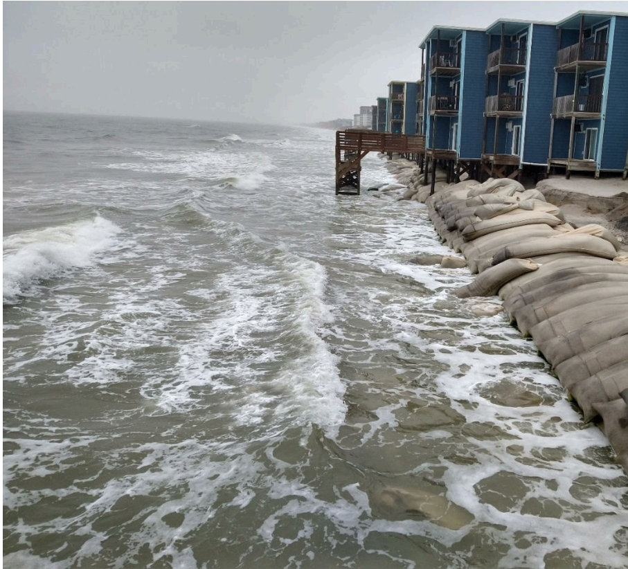
Figure 6: March 16, 2021 photo of the sandbags protecting the Topsail Reef Villas at high tide (looking south).
