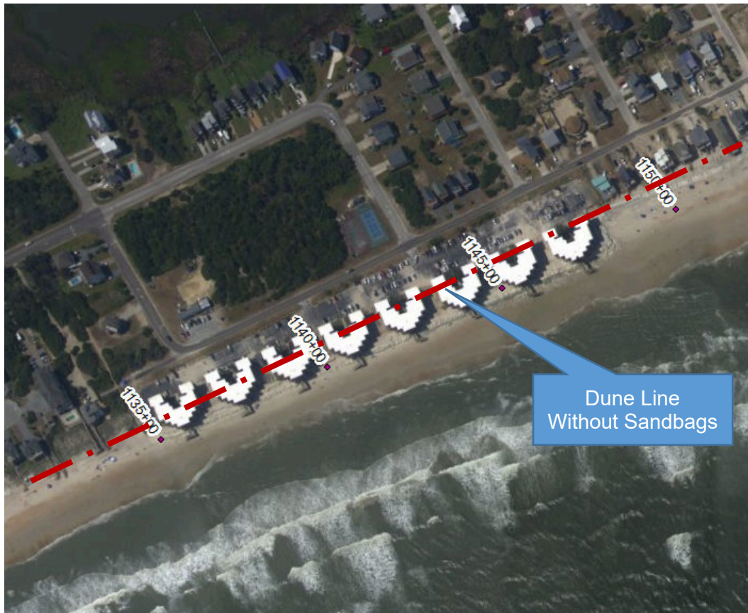
Figure 4: 2020 aerial with red dashed line showing where dune line would be without the sandbag protection.
