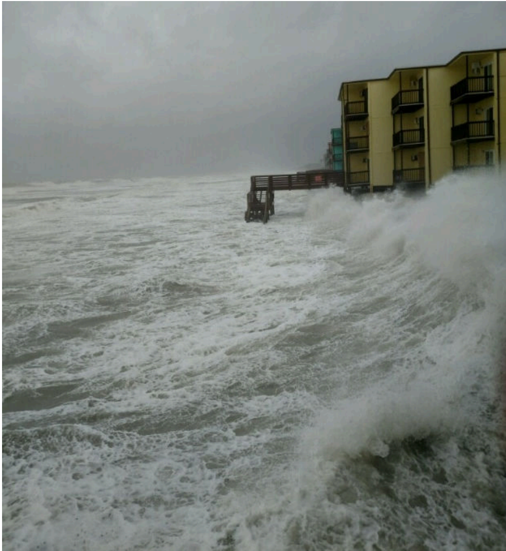
Figure 3: Hurricane Florence impacts on Topsail Reef Villas.
