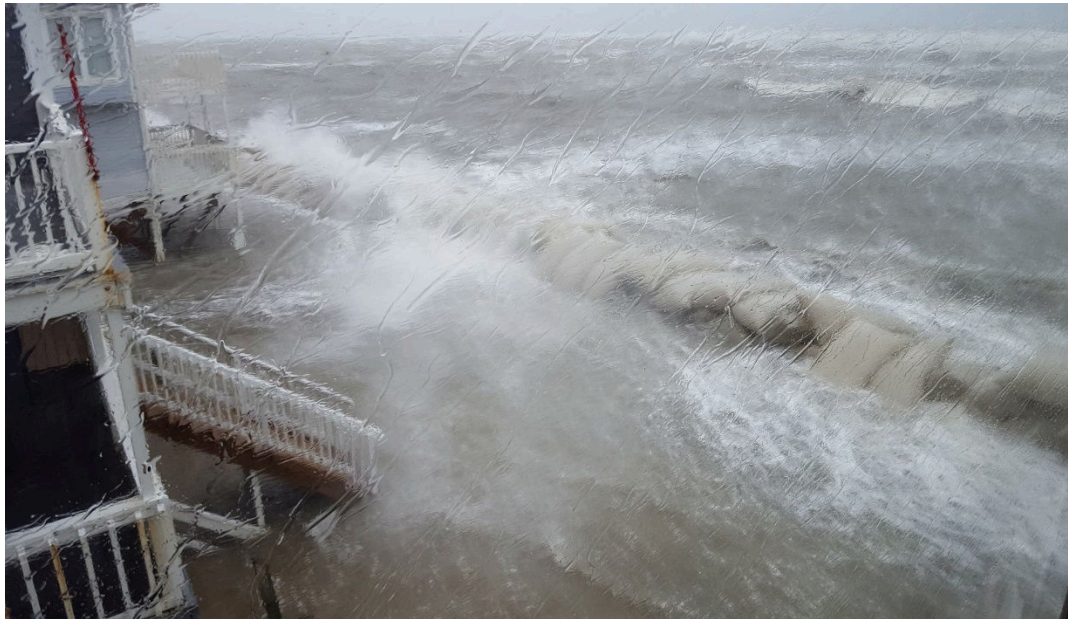
Figure 2: Hurricane Matthew impacts on sandbag revetment just to the north of Topsail Reef Villas.
