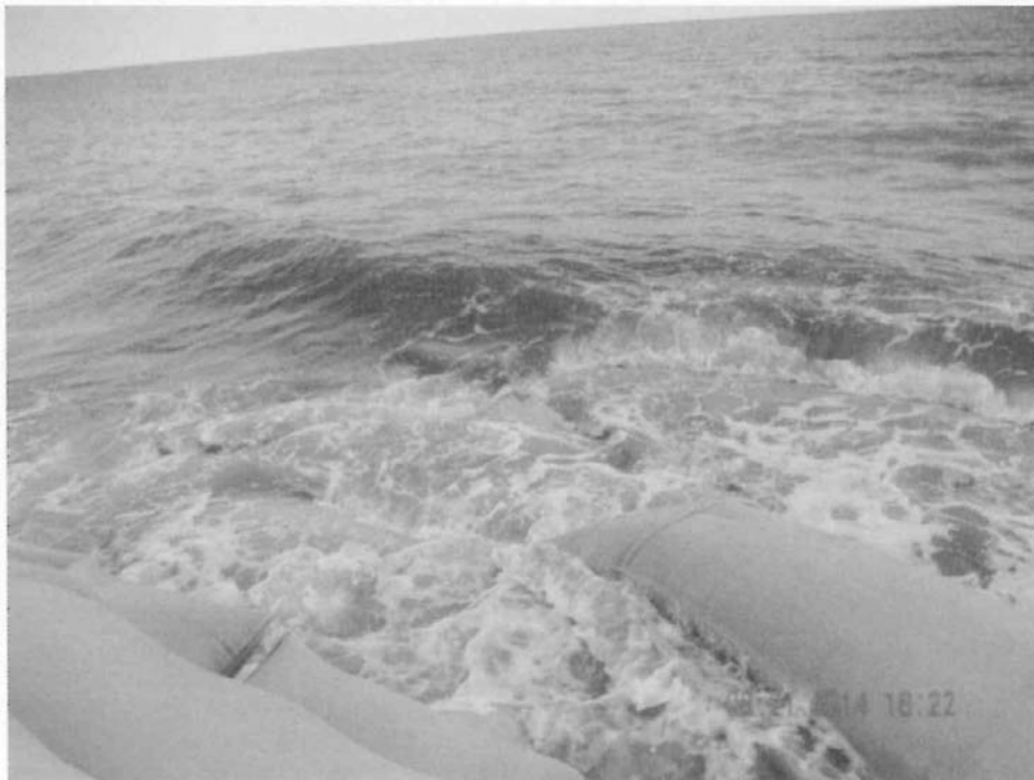
Photo 2 - Building 1 toe of revetment, August 21, 2014
