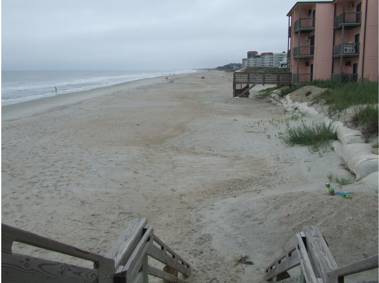
Photo taken by DCM staff on September 24, 2014, showing the erosion escarpment and existing sand bag structure in front of Building 8, Topsail Reef (looking south from Building 7).
