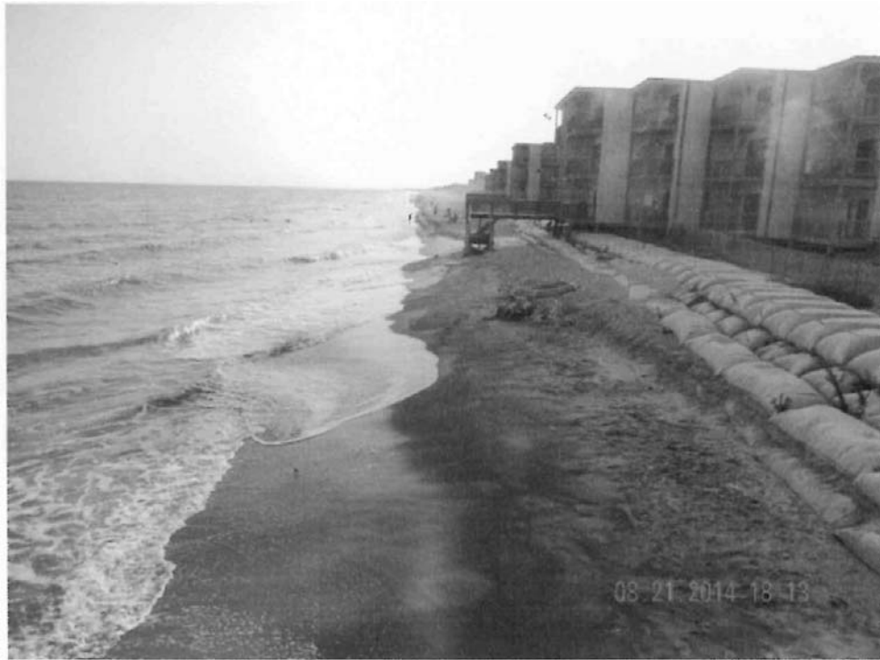
Photo 3 – At building 3 looking south at buildings 4 and 5, August 21, 2014
