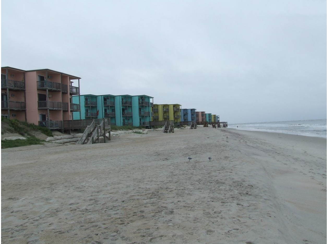
Photo taken by DCM staff on September 24, 2014, looking north showing the erosion escarpment and existing sand bag structures at Buildings 8-1, Topsail Reef (from left to right, respectively).
