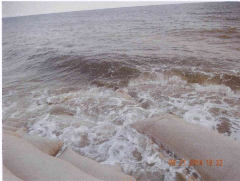
Photo 2 - Building 1 toe of revetment, August 21, 2014
