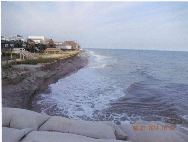
Photo 1 – Building 1 looking north, August 21, 2014
