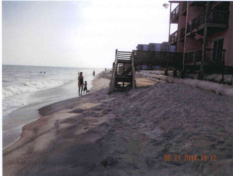
Photo 4 – At building 4 looking south at buildings 5 and 6, August 21, 2014
