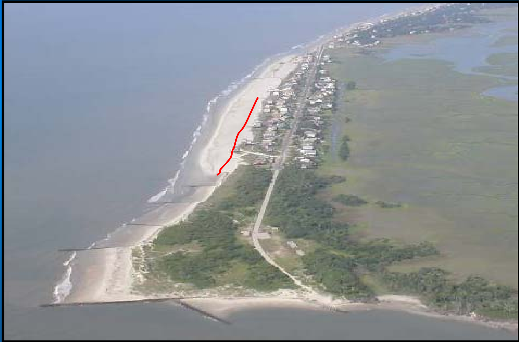
Photo: Construction of 2005 Renourishment
