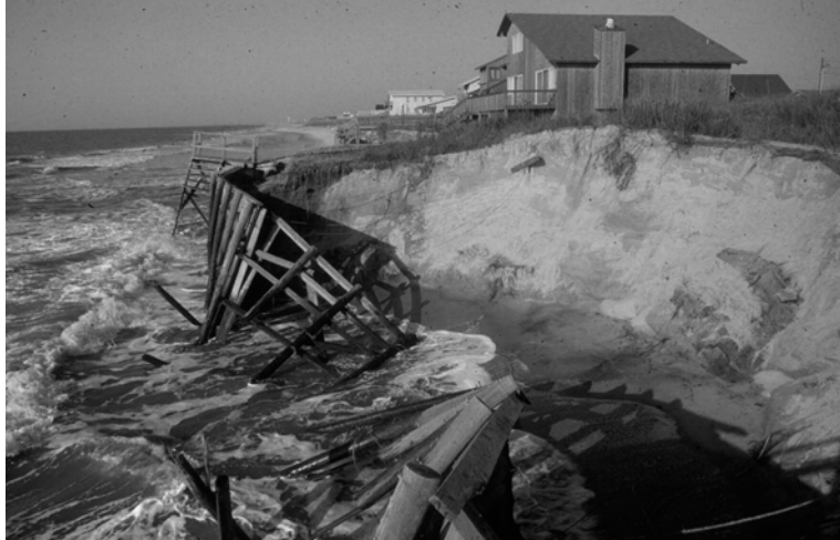
A vertical wall fails on Oak Island during the early 1980s.
