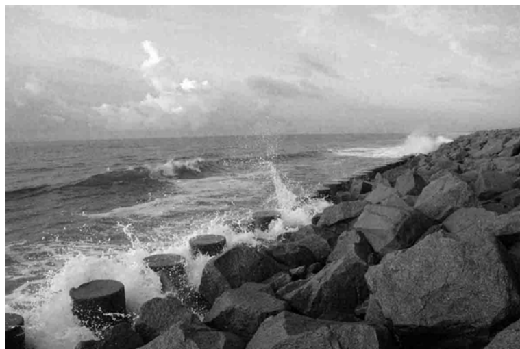
This stone revetment was built at Fort Fisher in 1996 by the Army Corps of Engineers to protect the civil-war era fort. It was the last revetment built in North Carolina.
