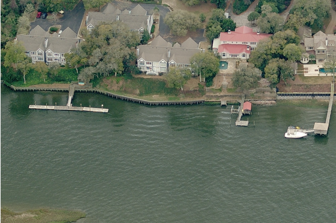
Figure 9: Estuarine shoreline erosion control structures near Charleston, SC. Many stretches of tidal creek shorelines in South Carolina have been armored with a variety of structures including wooden bulkheads and rock revetments.
