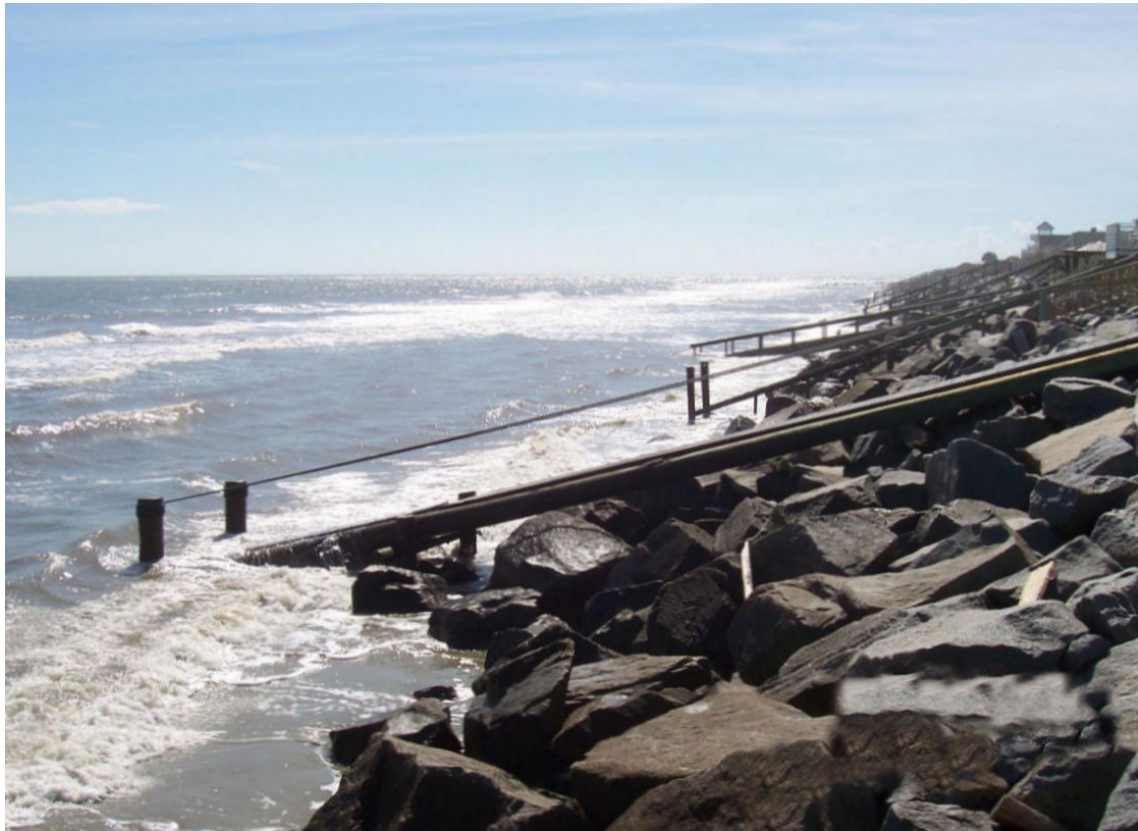
Figure 6: Revetment on Fripp Island, SC. Photo taken September 24, 2009.
