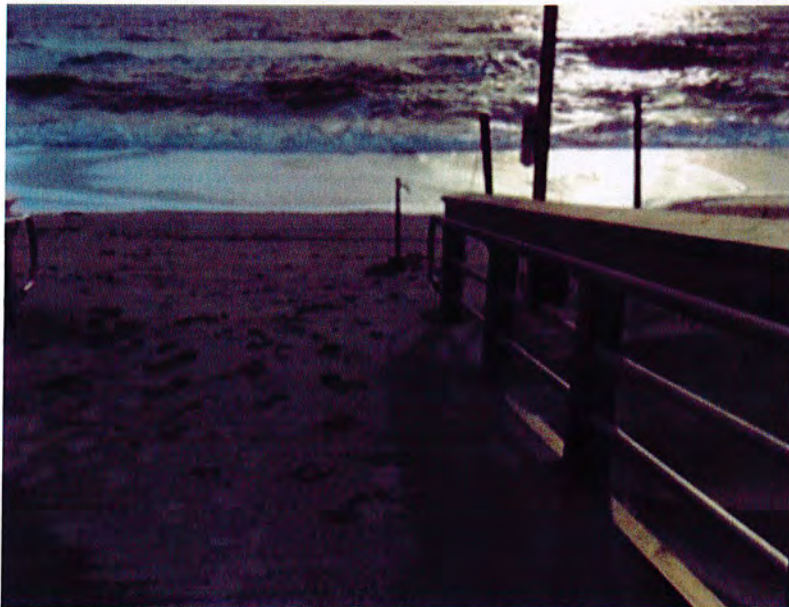
Photo taken on Oct. 28, 2015. Ramp from the Boardwalk in Carolina Beach. Note the metal water spigot is at the end of the ramp.
