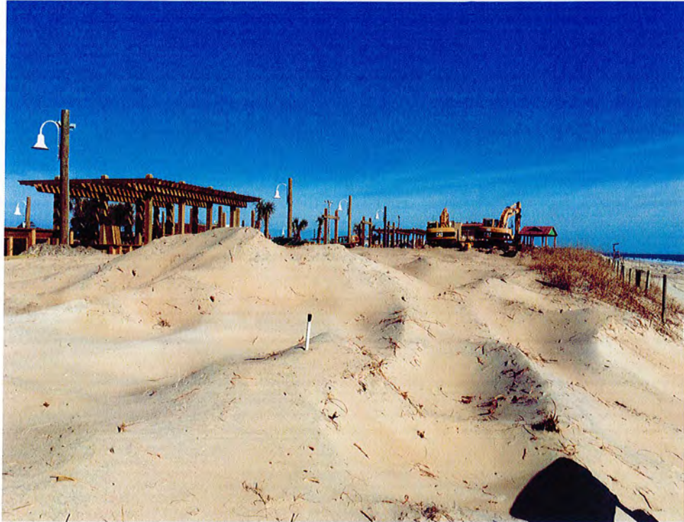
Feb 21, 2015 - Work in progress
