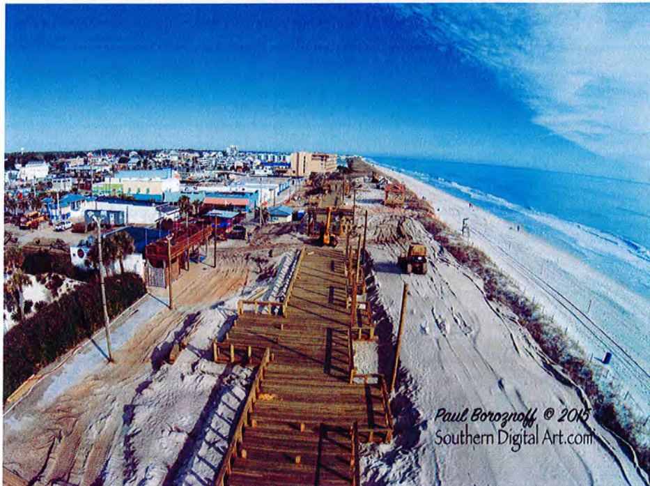
Jan 2015 - Aerial view of construction
