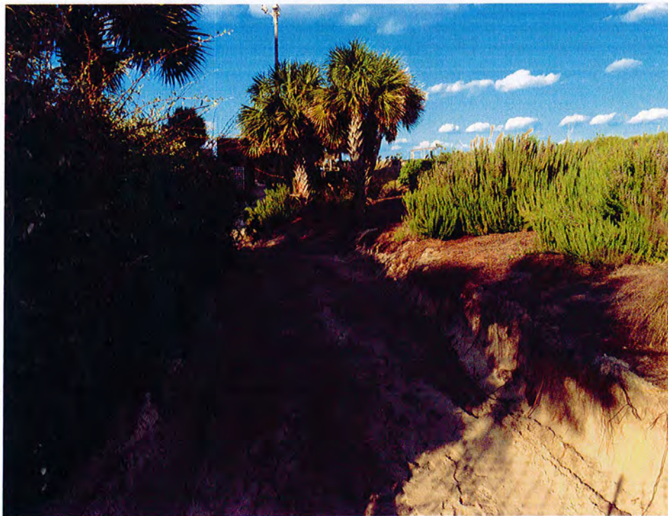
October 22, 2014 - First cut through the dunes and vegetation
