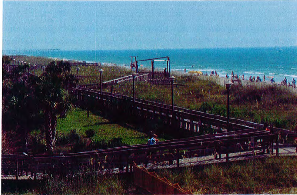
Boardwalk area looking north before work began on replacement
