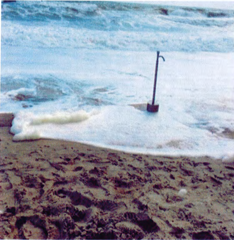
Sand and waves on end of Boardwalk ramp in Carolina Beach.
