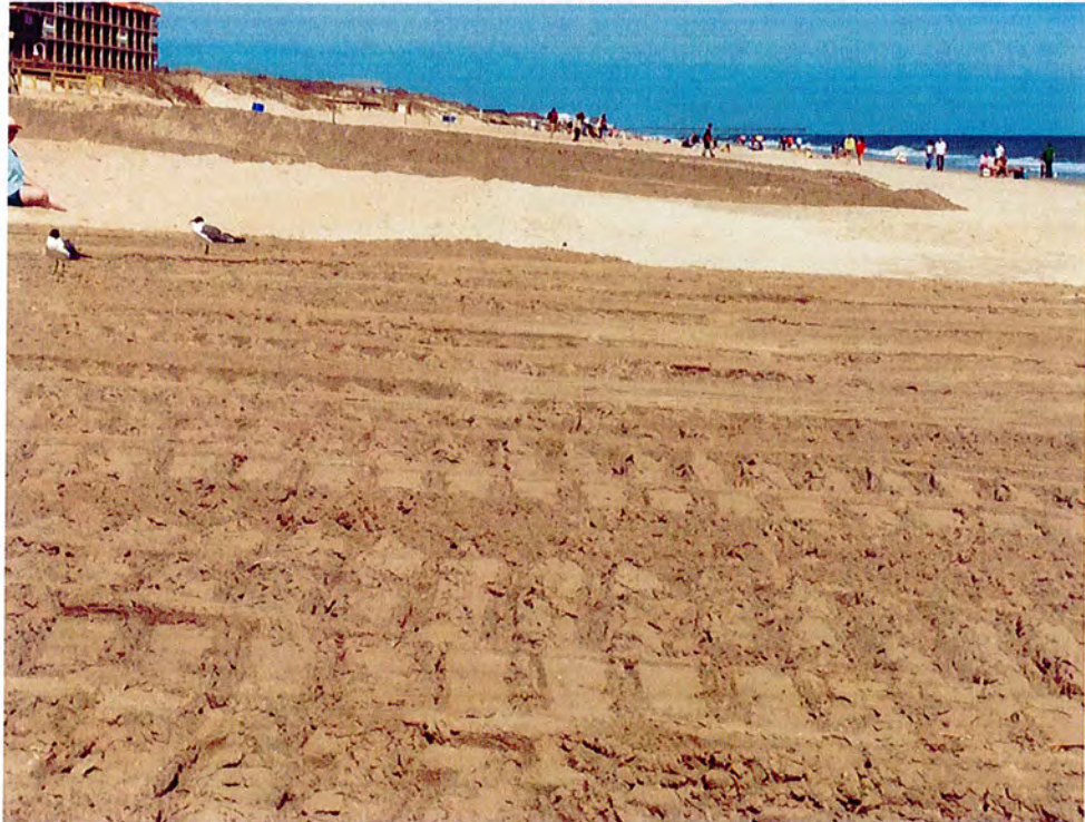
March 15, 2015 - Pushing sand onto beach
