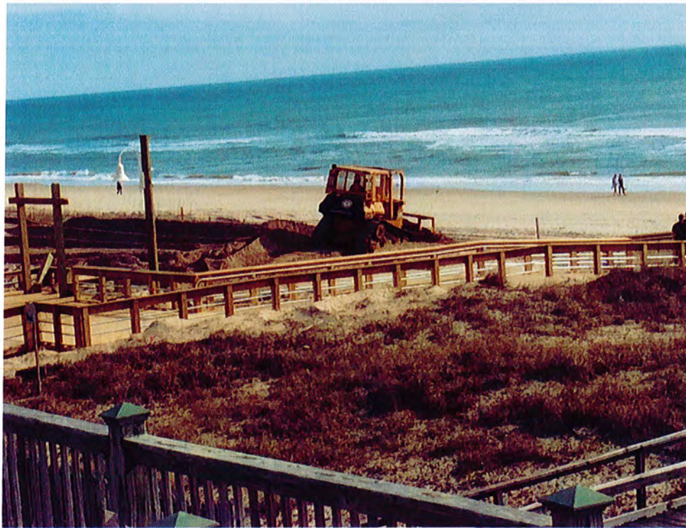
March 15, 2015 - Pushing sand onto beach
