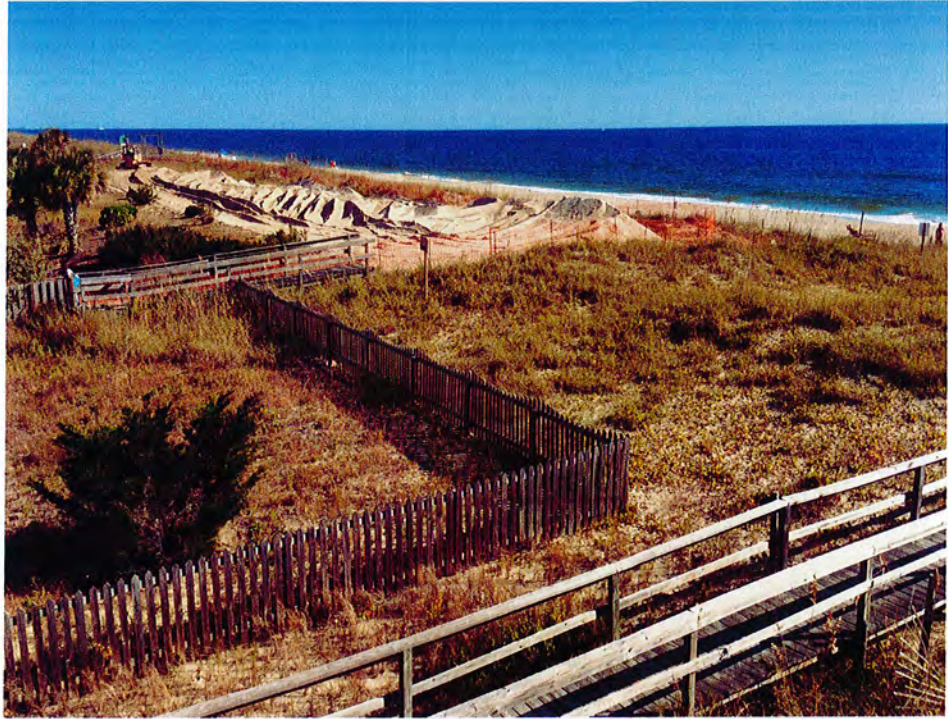
October 27, 2014 - Early stage of construction
