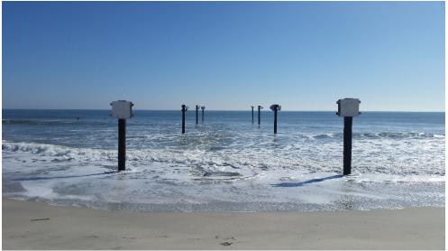
Fig. 3 Outfall buried and extended beyond the surf zone, and marked with warning signs
