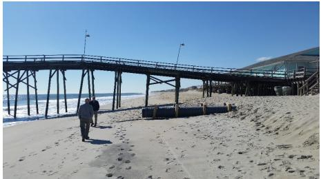
Fig. 2 Exposed outfall pipe and framing on an eroded beach
