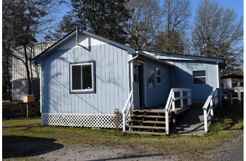
Figure 22. Reserve Northern Office
